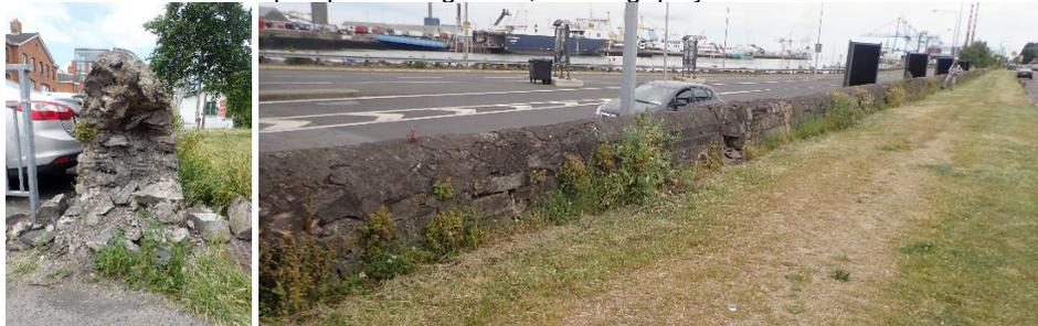
View showing breach in north-facing parapet, and view looking east along north-facing parapet from York Road
