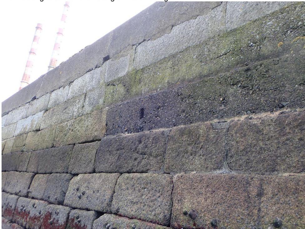
Detail view of north-facing elevation of harbour wall showing the stepped profile that is typical of the construction of the GSW.
