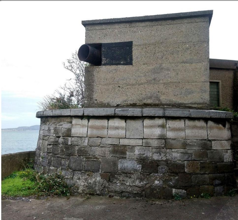
Photograph showing the former gun emplacement located , ADCO STR-03, above the harbour wall. The concrete structure built within the gun emplacement is thought to be a pillbox (guard-post) of twentieth-century date. Image courtesy of Cormac Lowth
