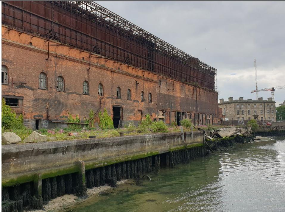
View looking south-southeast along current west-facing wharf of Pigeon House Harbour. The wharf is supported by a mass concrete quayside that was likely added to the original line of the GSW when constructing the generating station.
