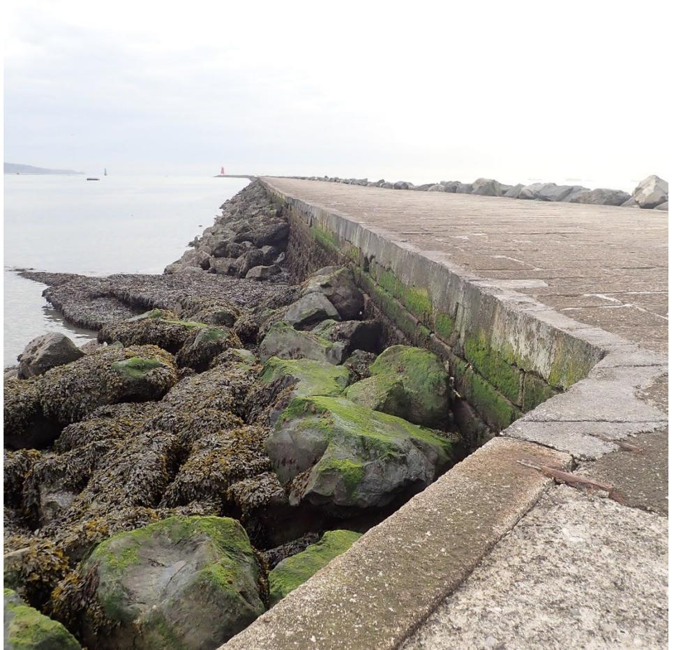
View looking east along GSW today just past White Bank Wharf Slipway ((DCIHR 19\_09\_011\_01). The rock armour protection placed at the base of the wall on the foreshore, and reaching the deck level on the south side are modern interventions
