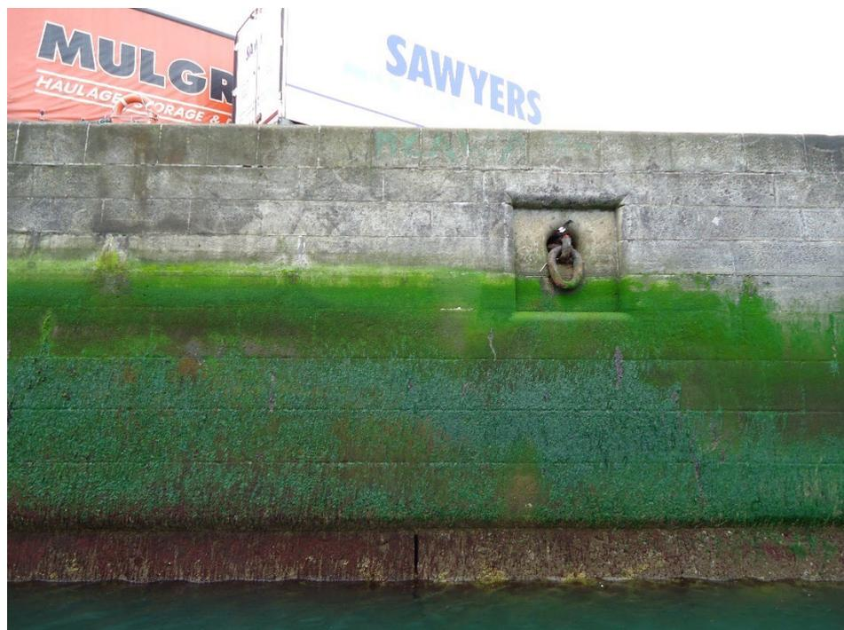
Photograph shows the top of two mass concrete foundation blocks and the join between both at the base of the image, with the granite ashlar coursing constructed above and a recessed mooring ring
