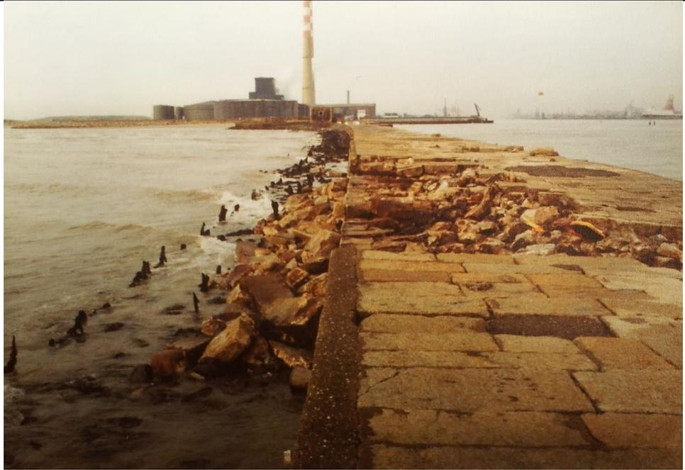
Photograph taken after the storm in 1981 shows damage to the GSW and a line of timbers off the south side, which appear to be the remains of 'The Piles'. Source: Dublin Port Company, Port Engineer
