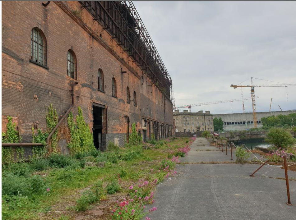
View looking south along the west-facing façade of the Electricity Works building, and the concrete quayside likely added to the original line of the GSW to facilitate the generating station
