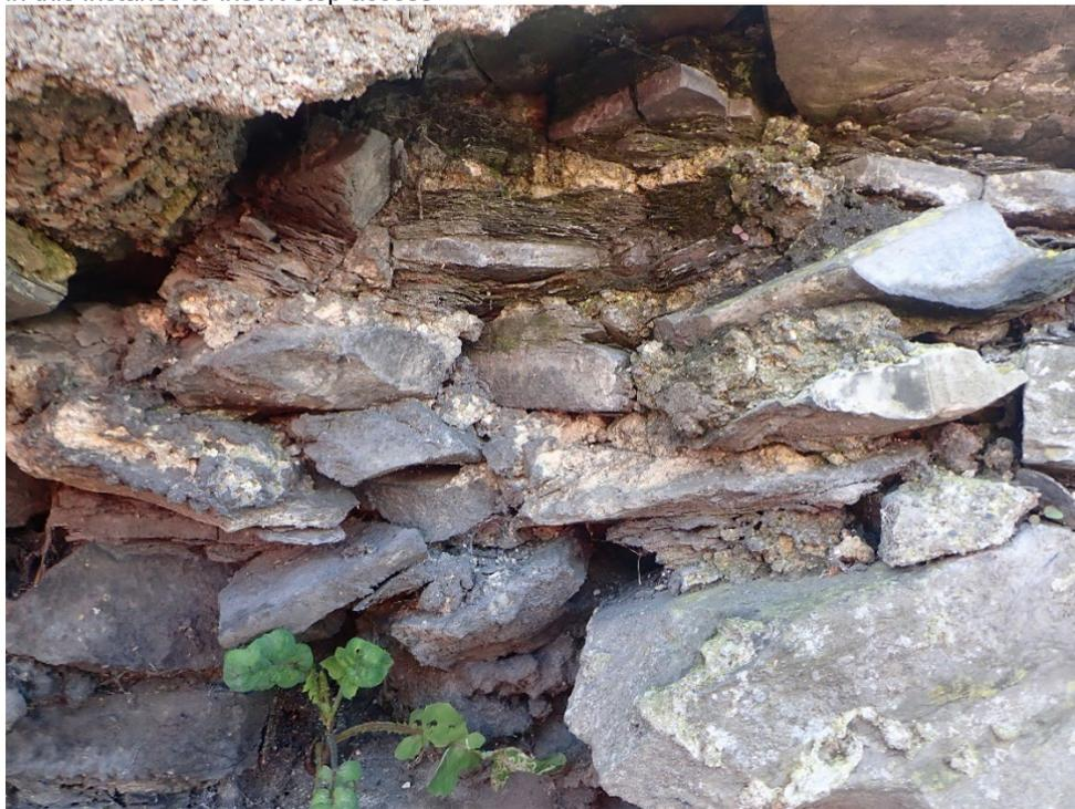
Detail showing fabric of the south parapet of the GSW in the MTL Yard where the wall core is exposed
