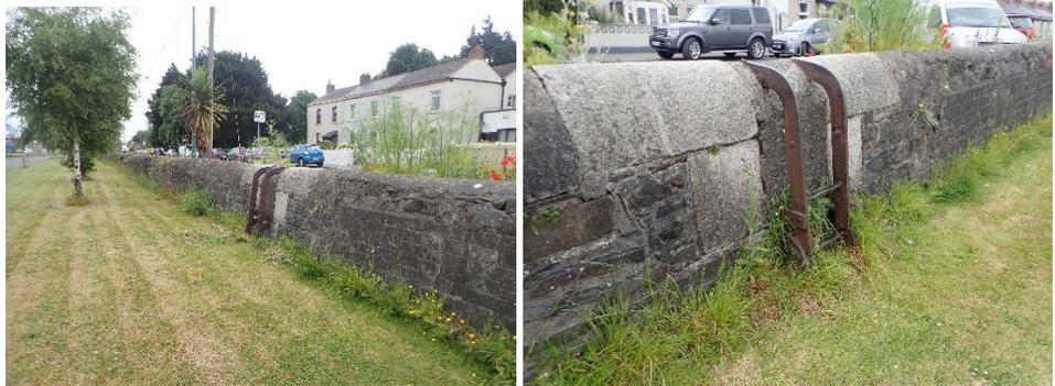
Two views of northern parapet looking south, showing quay wall ladder retained
