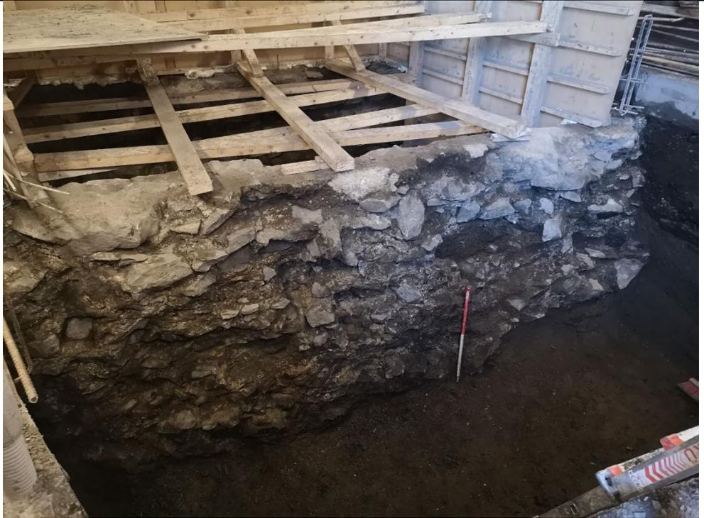
Excavated length of the former sea wall that lies under the Substation
