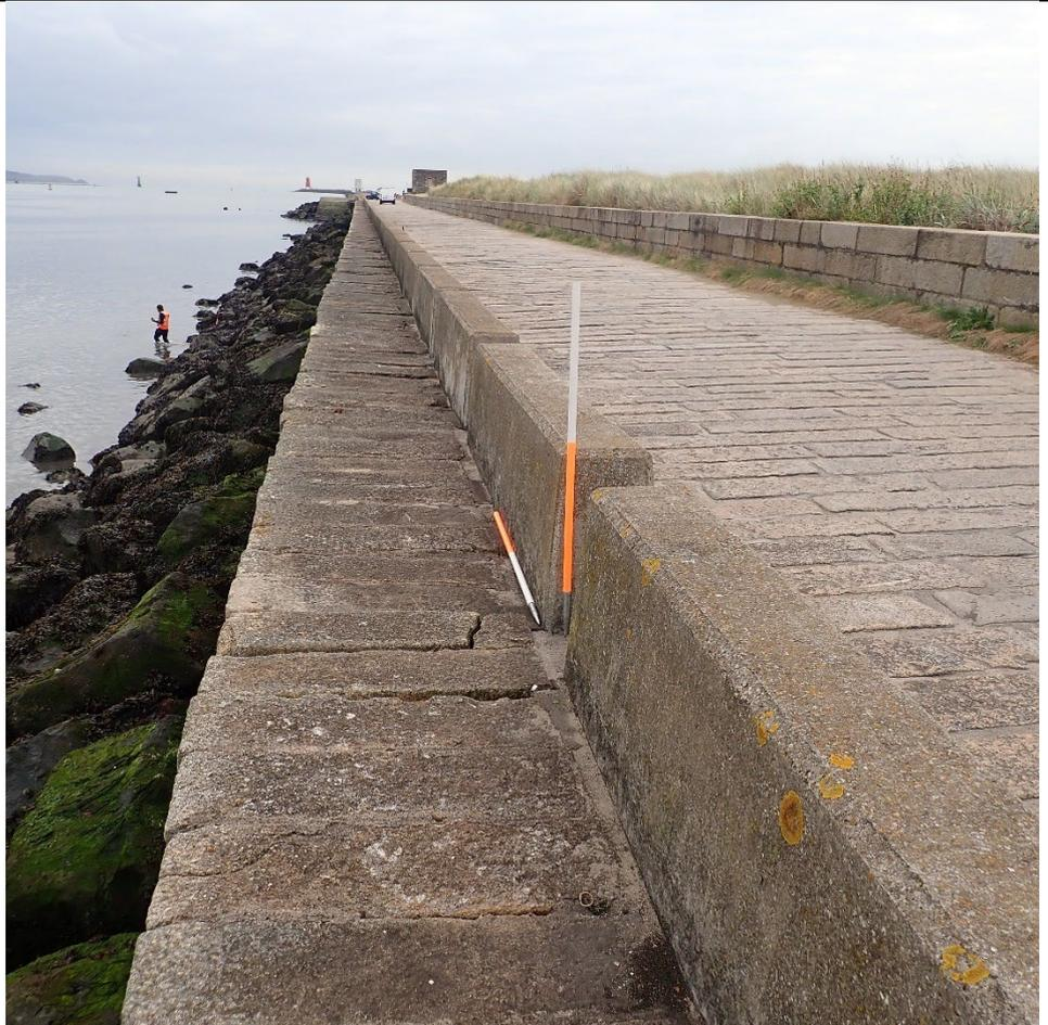
View looking east along GSW today alongside the Lifeboat House site (DCIHR 19\_09\_008\_01). The low concrete barrier supporting the vertical ranging rod is a modern addition
