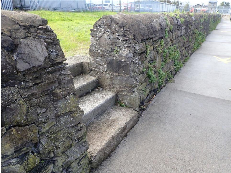
The south parapet of the GSW within the MTL Yard has been breached in several places, in this instance to insert step access
